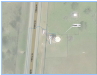
Plant 18 Paint and Rehab - Aerial
