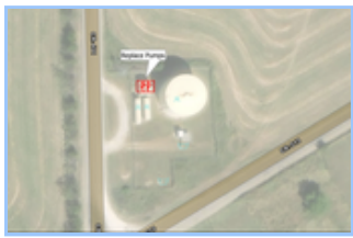
Plant 3 Pump Station - Aerial
