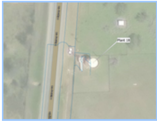
Plant 18 Pressure Tank - Aerial
