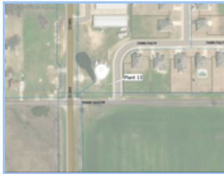
Plant 13 Paint and Rehab - Aerial
