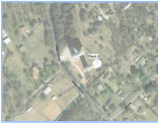
Plant 8 Paint and Rehab - Aerial
